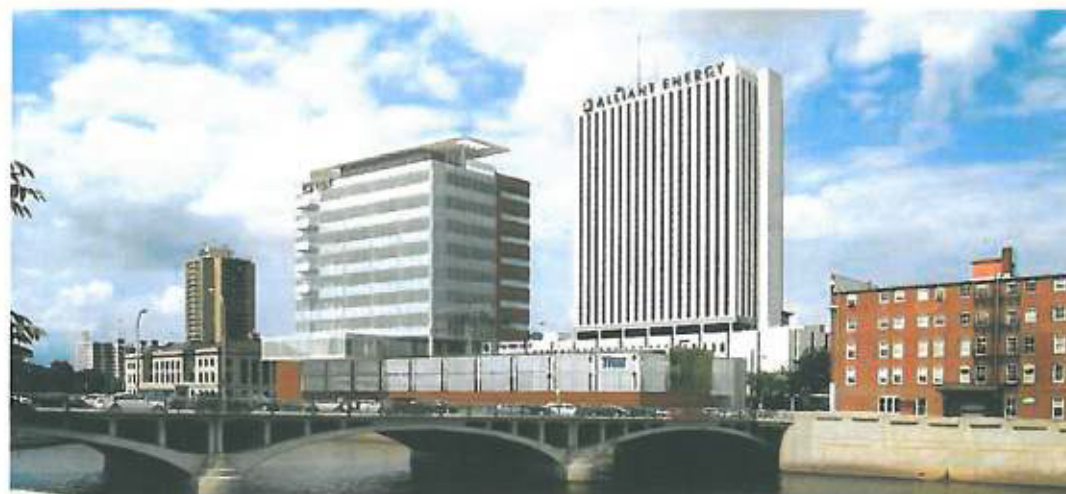
CSRT's new 11-story corporate headquarters in downtown Cedar Rapids was designed by OPN Architects and constructed by Ryan Cos. US Inc. The building is expected to be ready for occupancy in the spring of 2016. Design features include a cantilevered office component over the Cedar River and 300 feet of the new Cedar Rapids flood protection system.
